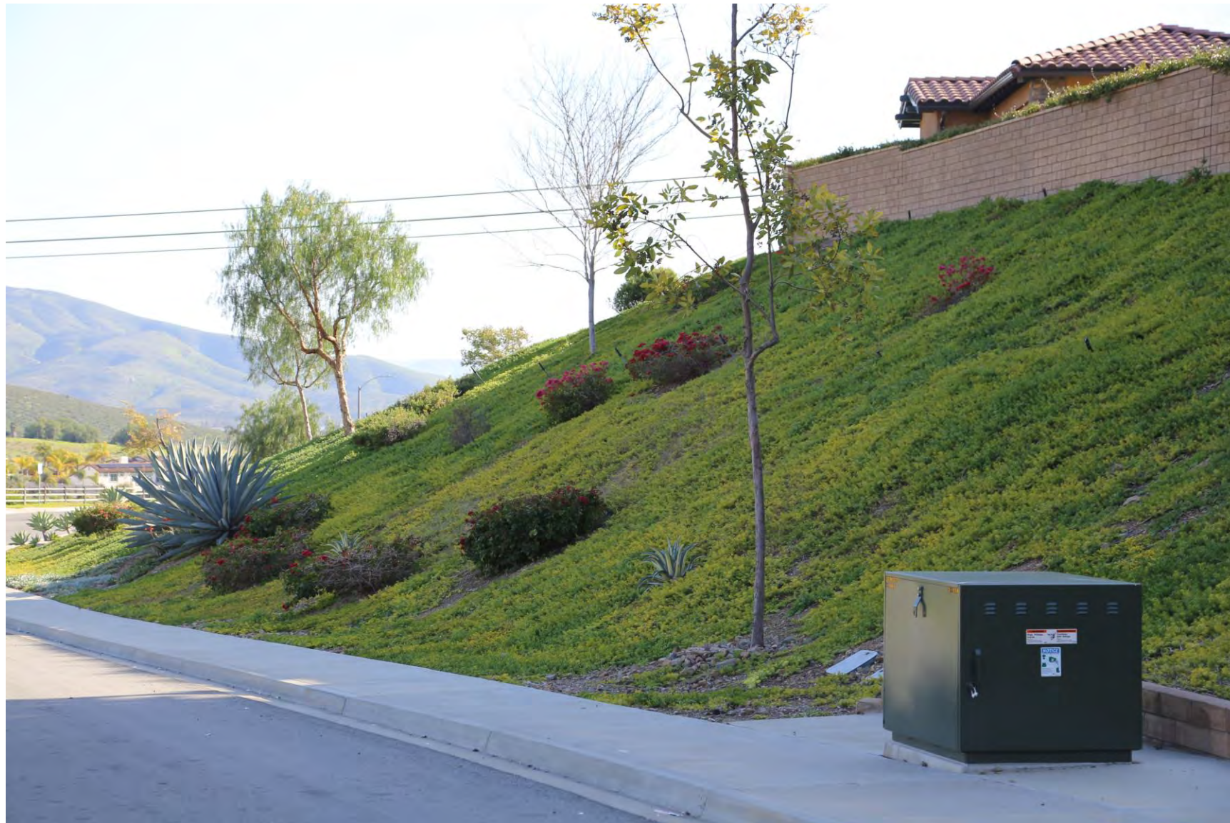
Large slope to sidewalk; Ground cover protects sidewalk and prevents erosion. Chula Vista
