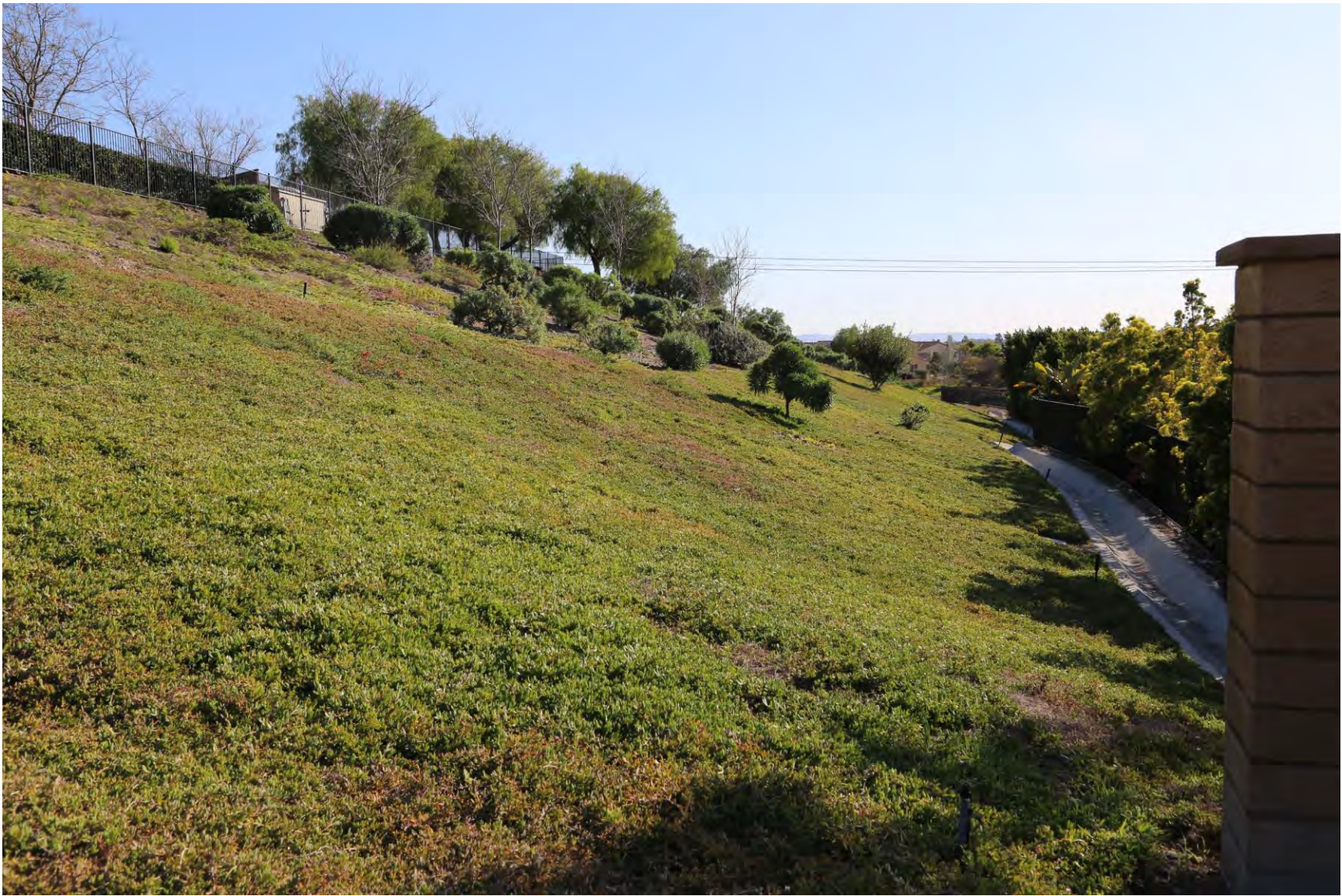
Large slope, trees, shrubs, ground cover grows to the swales preventing erosion runoff. FMZ compliant. Chula Vista
