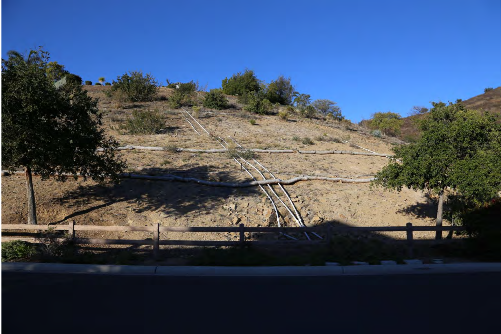
Hydroseed failed, bare ground etc
