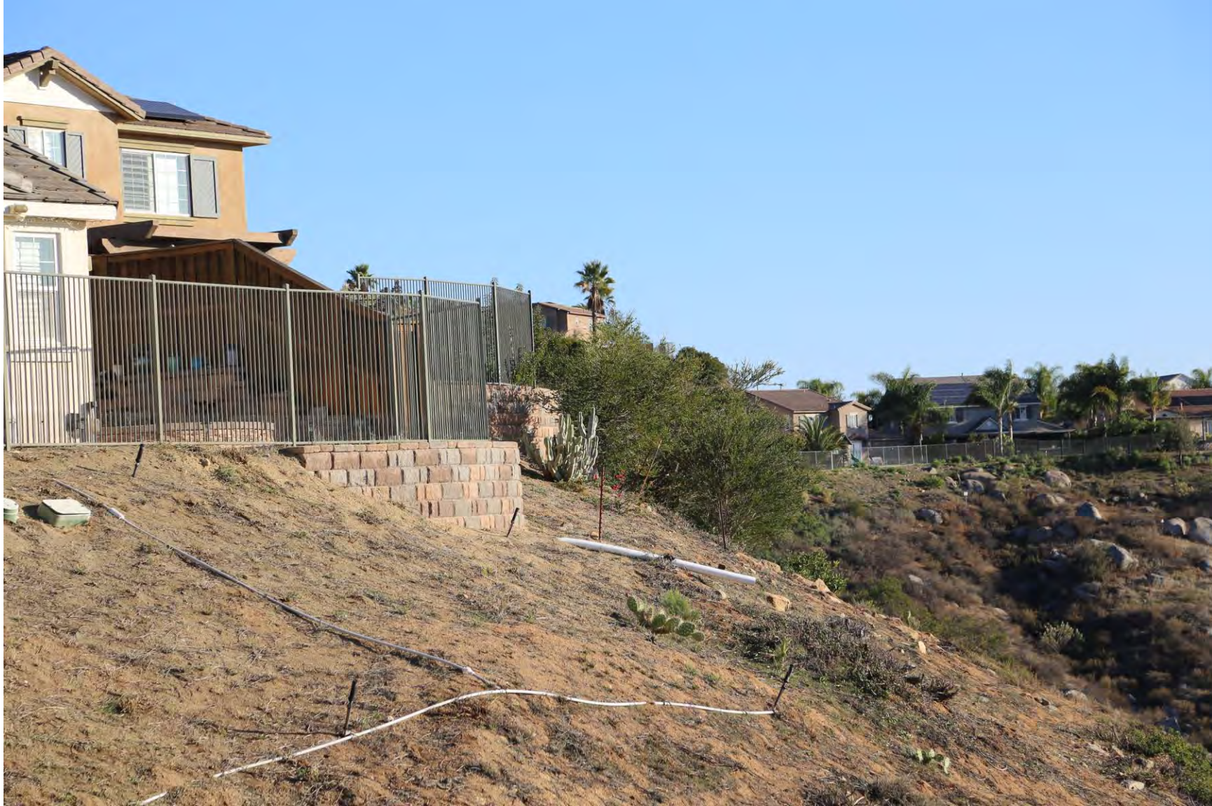
Exposed ground in FMZ, fence not cleared 18"
