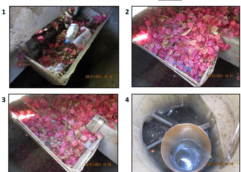
Photos #1-3: Remove accumulated leaf debris and trash from filter inserts.
